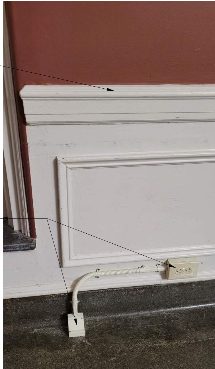
PHOTO 4 | TYPICAL WALL CONDUIT
